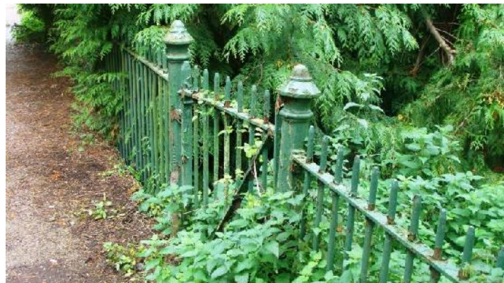
Picture 16. Good quality robust historic railings in need of minor repainting/refurbishment.
