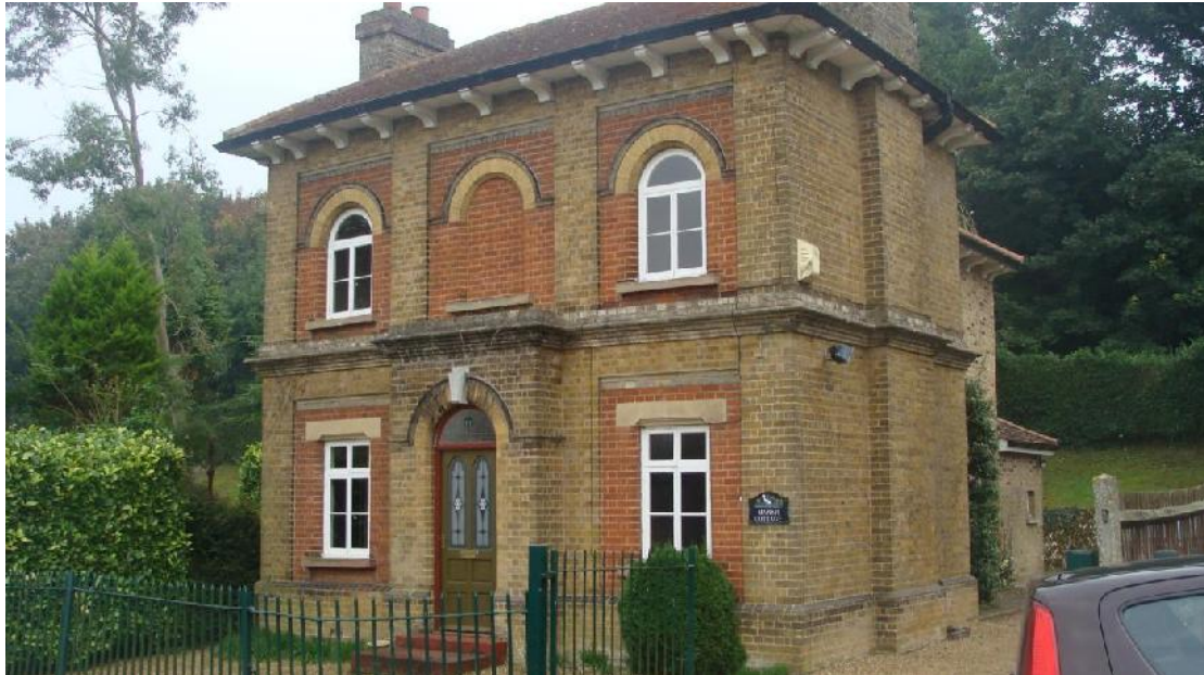
Picture 10. Marsh Cottage, former engineers house associated with the adjacent pumping station.
