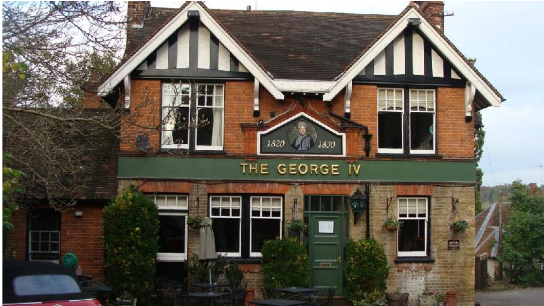
Picture 12. The George IV PH. A late 19th/early 20th century building of quality with many architectural features worthy of preservation through normal development control.
